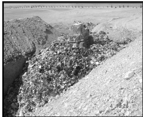
Figure 2. Trench method of waste disposal at Ma'an Landfill site.
