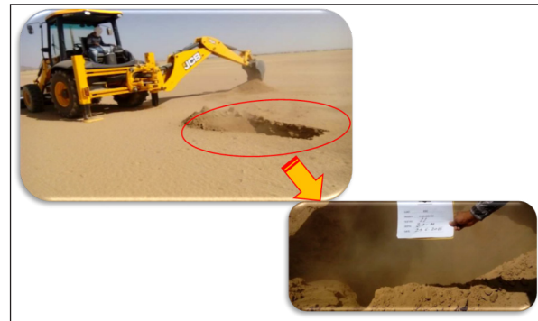
Figure 5. Excavation process of test pits in the study area
