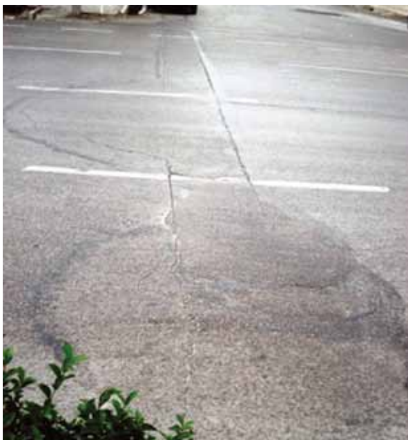
Figure 13: Crescent and round shaped subsidence in risky area with high distribution density of Qanat
