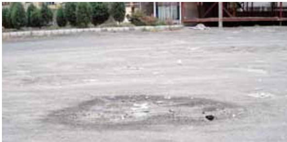
Figure 12: Round shaped subsidence formed in high-risky cells in potential map
