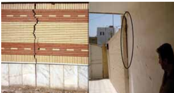
Figure 5: A crack in the wall of a building (left part) and tilting a wall (right part) on Andisheh Street west of Mashhad city (Hafezi Moghaddas et al., 2012)
