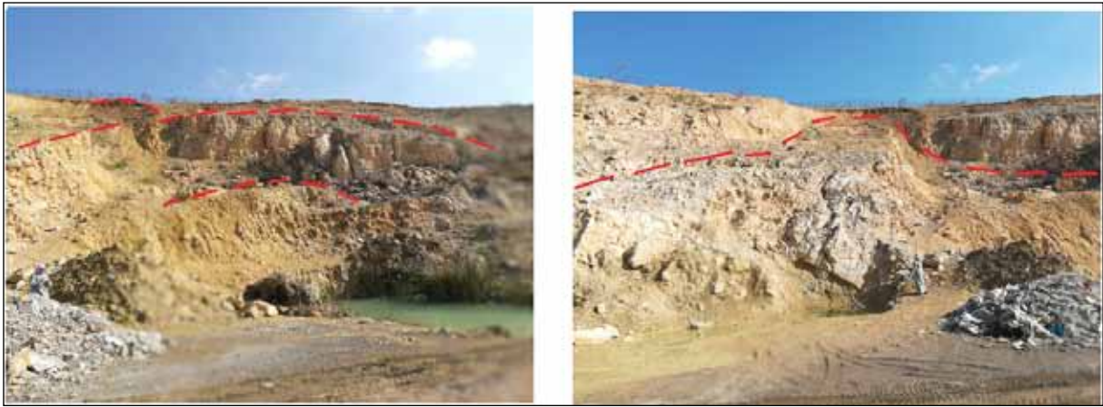
Figure 35. The outcrop shows the circular failure in station-9.
