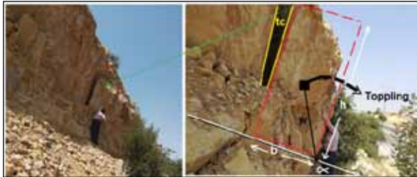
Figure 25. Toppling failure; tension crack (tc) acts as back release surface in station-5.
