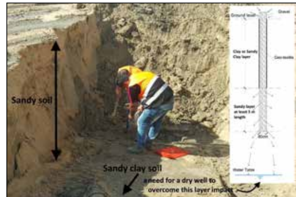
Figure 2. A real photo taken during the excavation for a stormwater pond depicting the need for dry well technique to penetrate a low permeable layer
