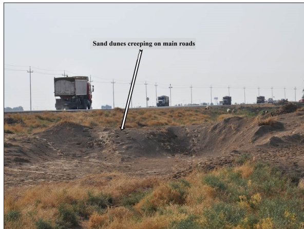
Figure 6. The encroachment of sand dunes on land roads
